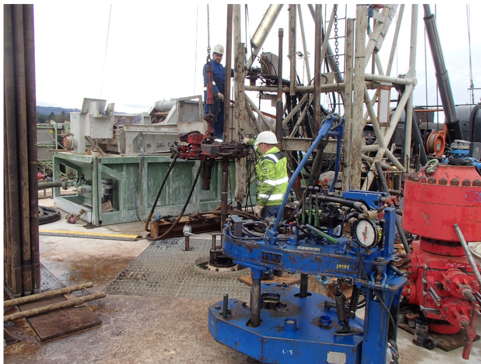
Running 2 7 / 8 inch tubing into the Anshof-3 well with the RED W-101 workover rig in preparation for testing operations. Source ADX
