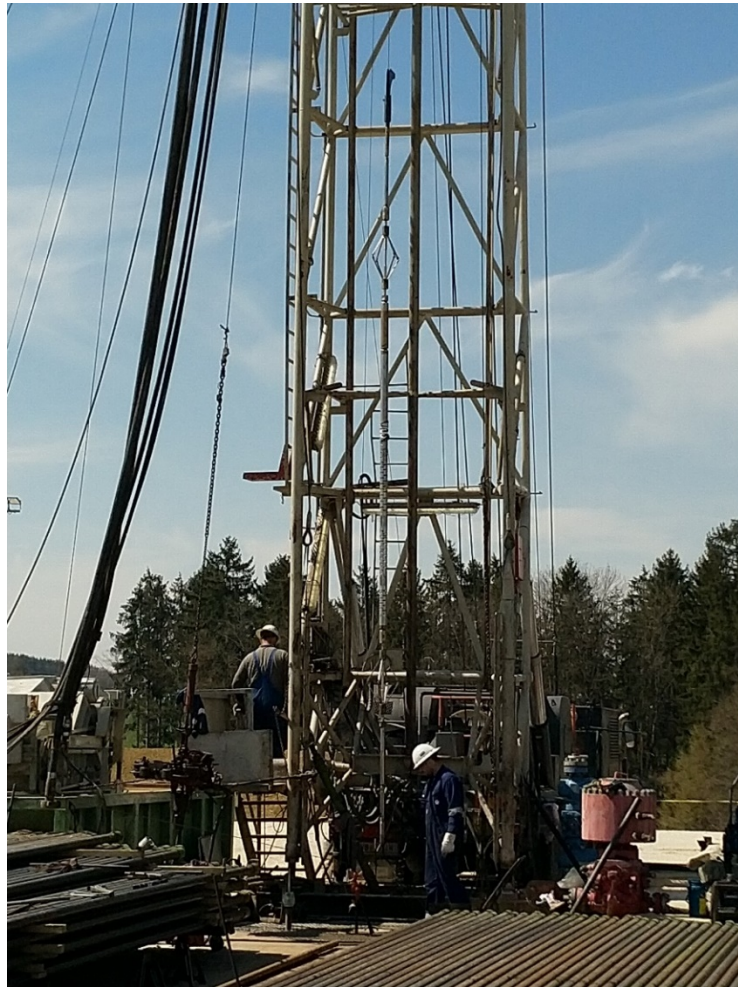
Running a cement bond survey to check well integrity of the Anshof-3 well with the RED W-101 workover rig in preparation for testing operations. Source ADX
