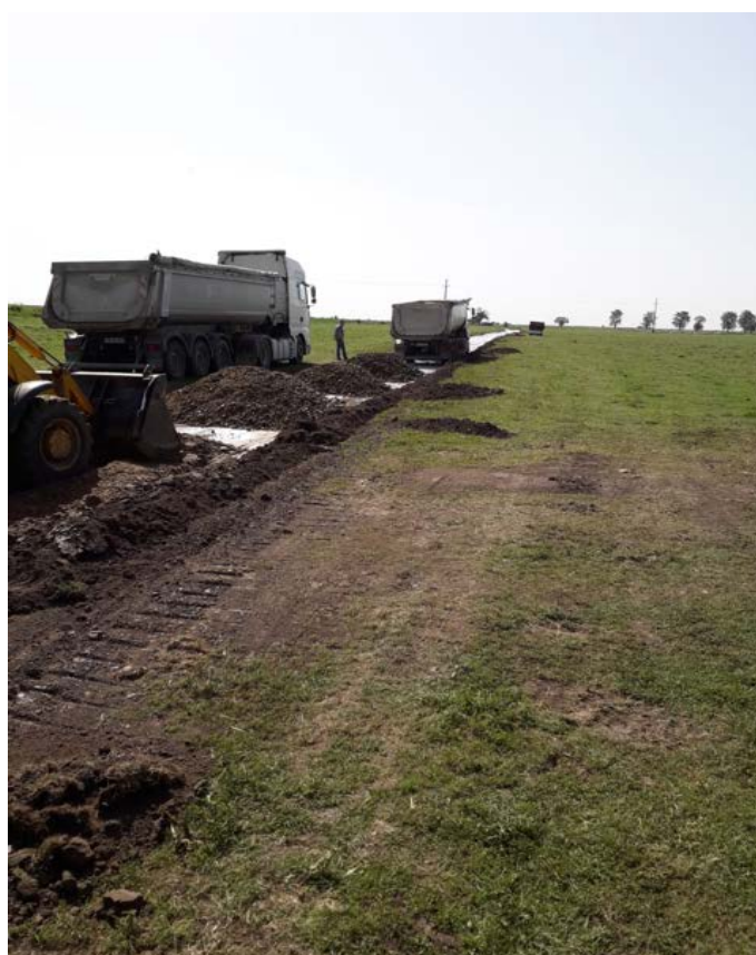
Iecea Mica 1 well road construction and membrane installation
