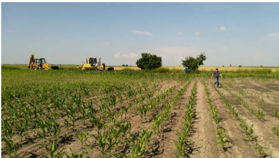
Iecea Mica-1 Well Access Road Construction across agricultural land
